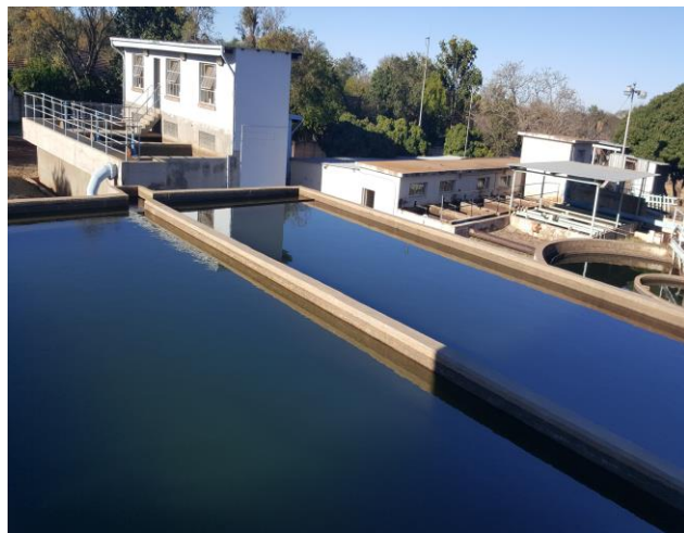
Bela- Bela Water Works
